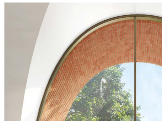
Close up of vaulted ceiling and windows.
